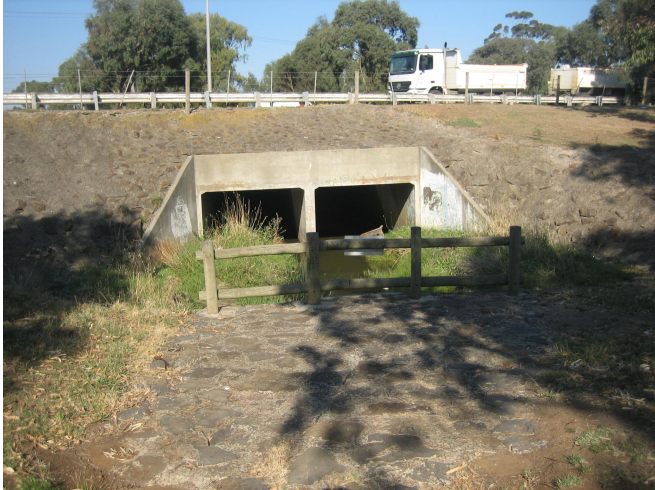
Figure 4: Existing structure downstream of Keilor Park Recreational Reserve Site
